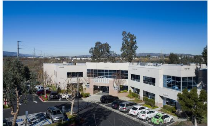
Campus parking and building access
